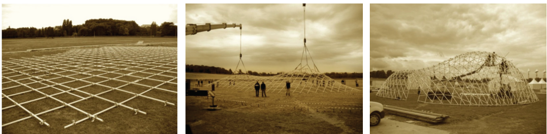
Figure 1 – 300 m 2 gridshell structure hosting the forum during the Solidays festival (2011) in Paris (France). Here, buckled beams shape a roof and provide mechanical robustness to the structure. Reproduced from du Peloux et al. (2013).
